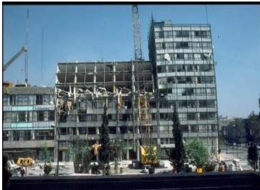
Fig. 4.9.1 Pounding of adjacent buildings in Mexico City (1985) due to SSI
