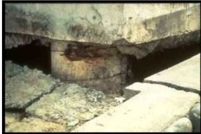
Fig. 4.8.3 Example of damage at the pile-cap connection
