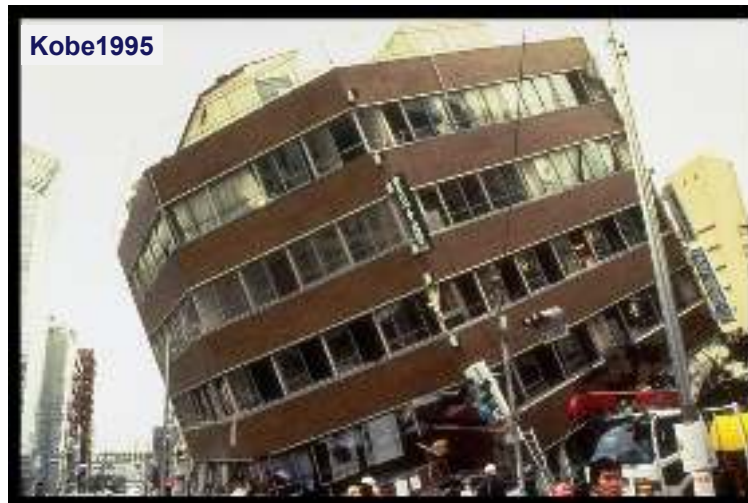
Fig. 4.5.1 Example of damages to a building caused by liquefaction of the foundation soil
