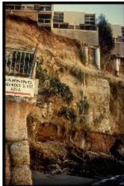
Fig. 4.6.2 Example of slope instability affecting constructions (Loma Prieta, 1989)
